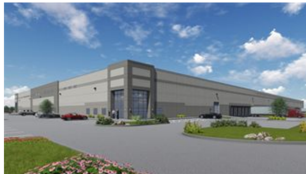
Becknell Industrial, Mount Comfort, IN (acquisition)
