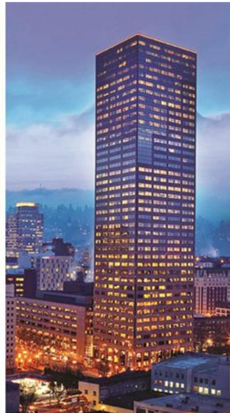
US Bancorp Tower, Portland, OR
